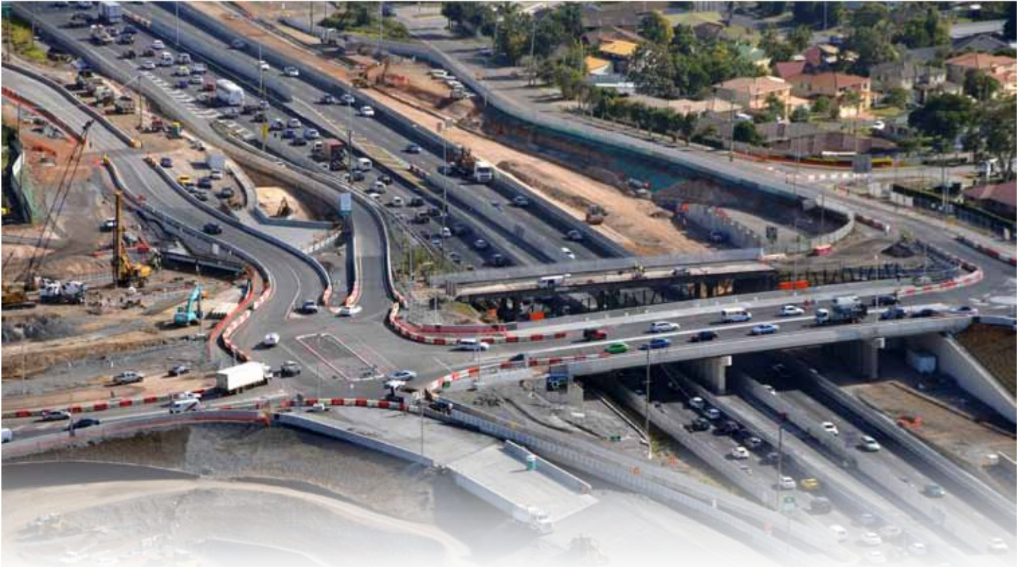
The new Loganlea Road overpass bridge is now open to traffic, with one lane operating in each direction.
